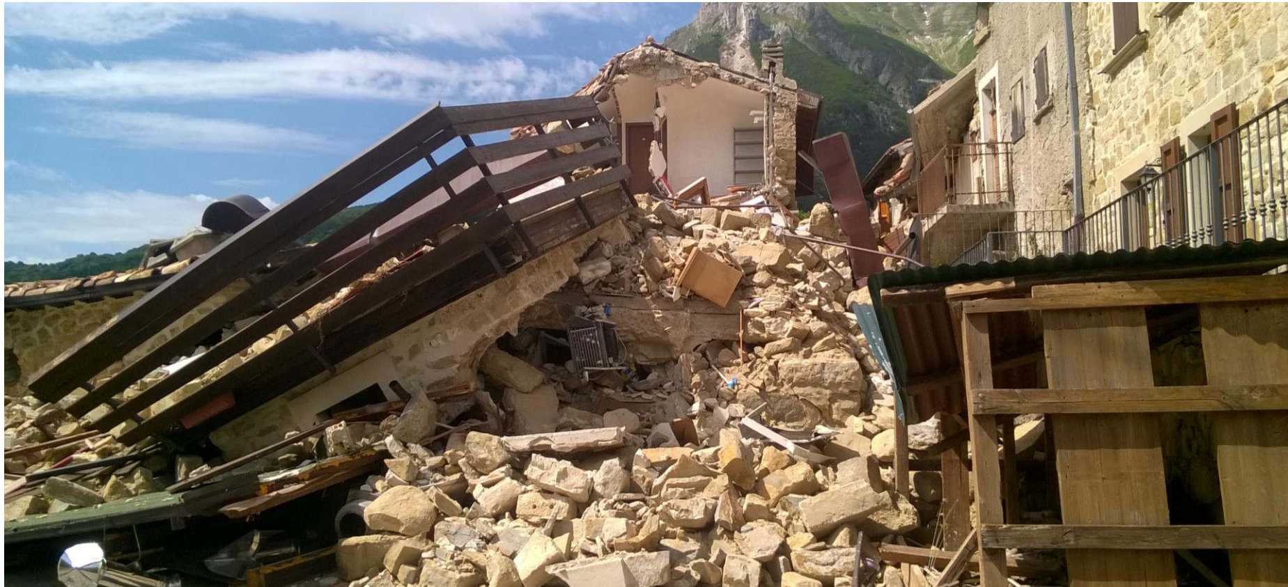
Montegallo, Frazione Colle
