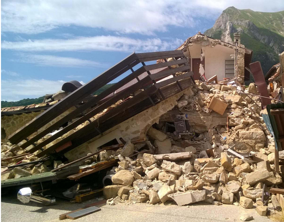
Montegallo, Frazione Colle
