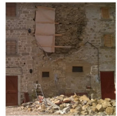
Montegallo, Frazione Colle
